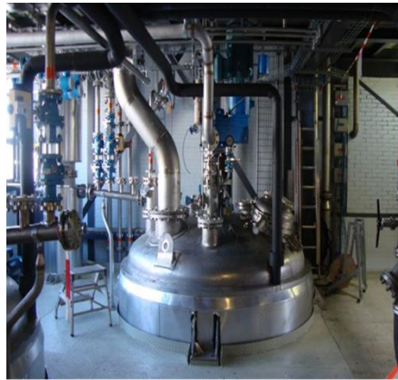
16 m 3 Hastelloy batch reactor, up to 16 bar,
