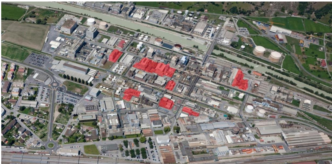
Backward integrated site in Visp, Switzerland, with complex multi-purpose plants, broad technology portfolio, and integrated waste management facilities
